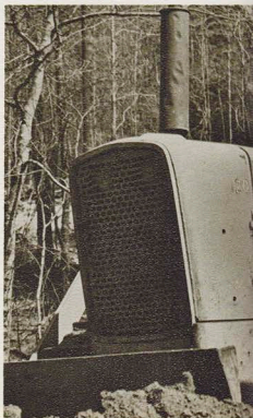
"Cat" at work on road.
